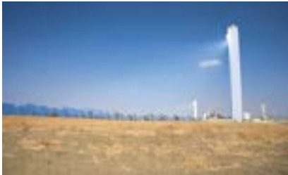
10MWe Direct steam solar tower receiver
