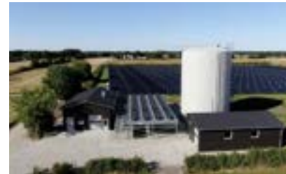
2.5 MWth integrated heat pump system
