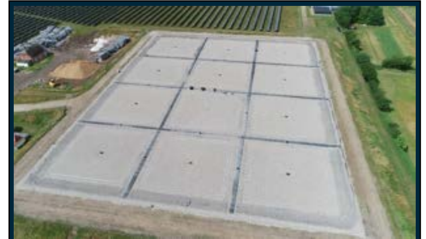
Pit Thermal Energy Storage in Marstal
