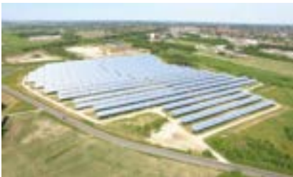
16.6 MWth combined CSP and ORC plant
